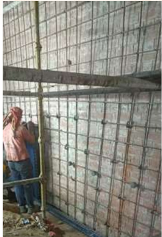
Step-3:- Reinforcement Binding for Jacketing on Brick Pier at Nehru Nagar Flyover (RoB)
