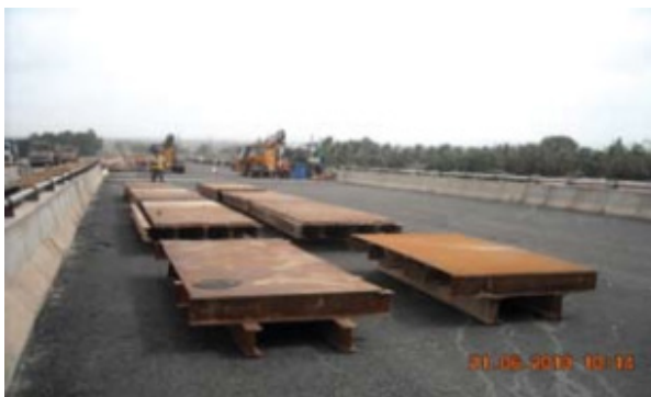
Photo 8 - Load testing by Static Method
