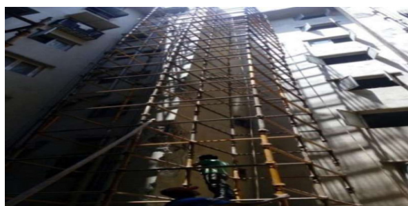
Fig: - Scaffolding Erection
