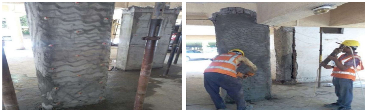
Fig: - Treatment to concrete core for strength improvement
