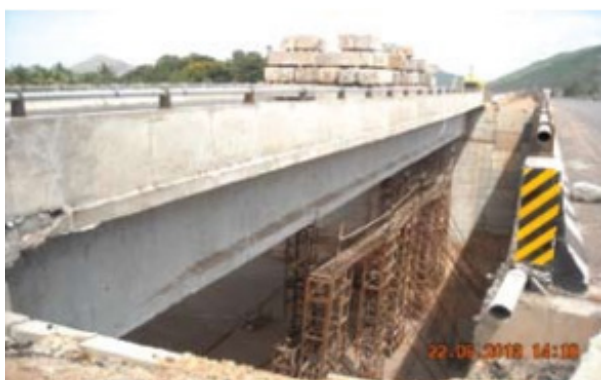
Photo 9 - Load Testing by Static Method - a Closeup of Loads
