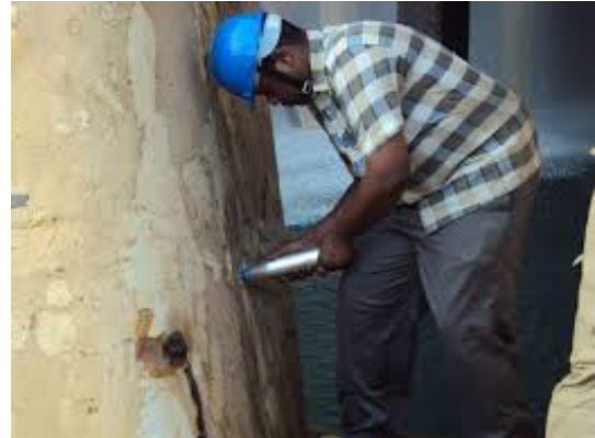
Fig: - Putty work on RCC wall
