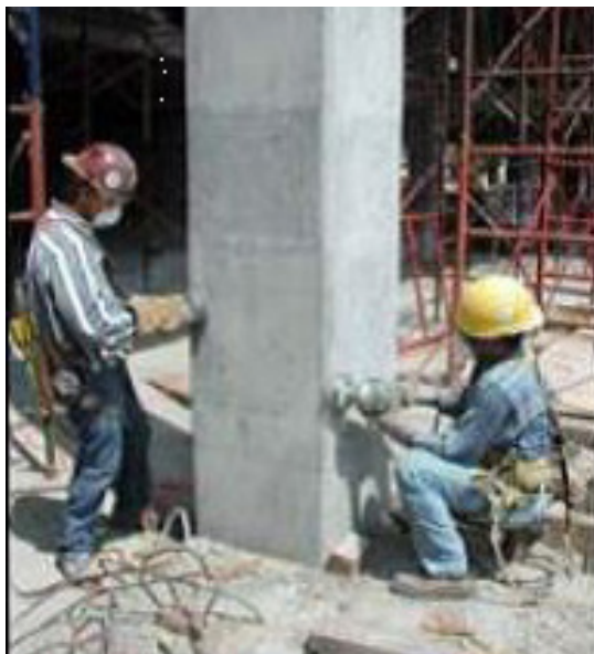
Fig: - Surface Preparation of RCC Column
