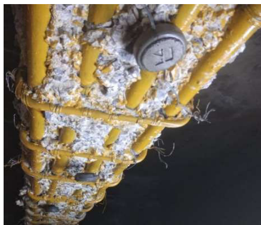
Step-5:- Fixing Sacrificial Galvanic Anode on Reinforcement at Nehru Nagar Flyover (RoB)
