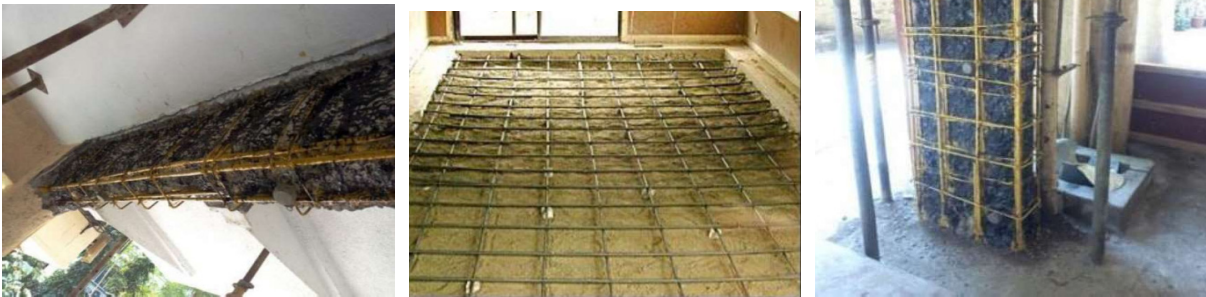
Fig: - Provision of additional reinforcement in Column, Beam and Slab
