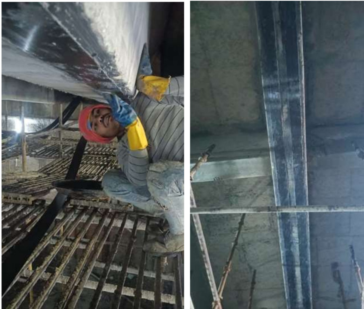
Step-7:- P/F Carbon Laminate on RCC Girder at Nehru Nagar Flyover (RoB)
