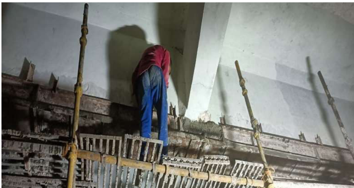
Step-6:- P/F Shuttering for Micro Concrete repair on RCC Girder at Nehru Nagar Flyover (RoB)
