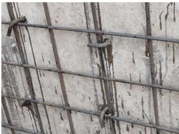
Step-4:- Shear anchoring to fix reinforcement on Pier at Nehru Nagar Flyover (RoB)
