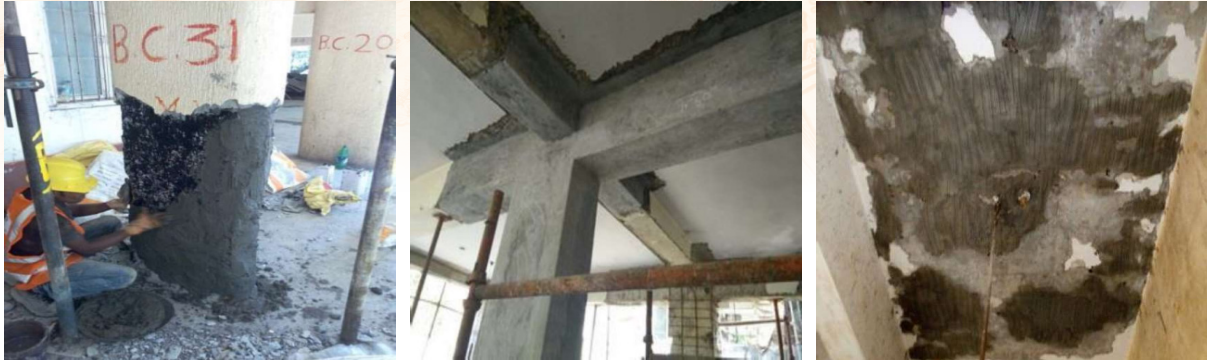
Fig: - Modified Mortar work on Column, Beam and Slab
