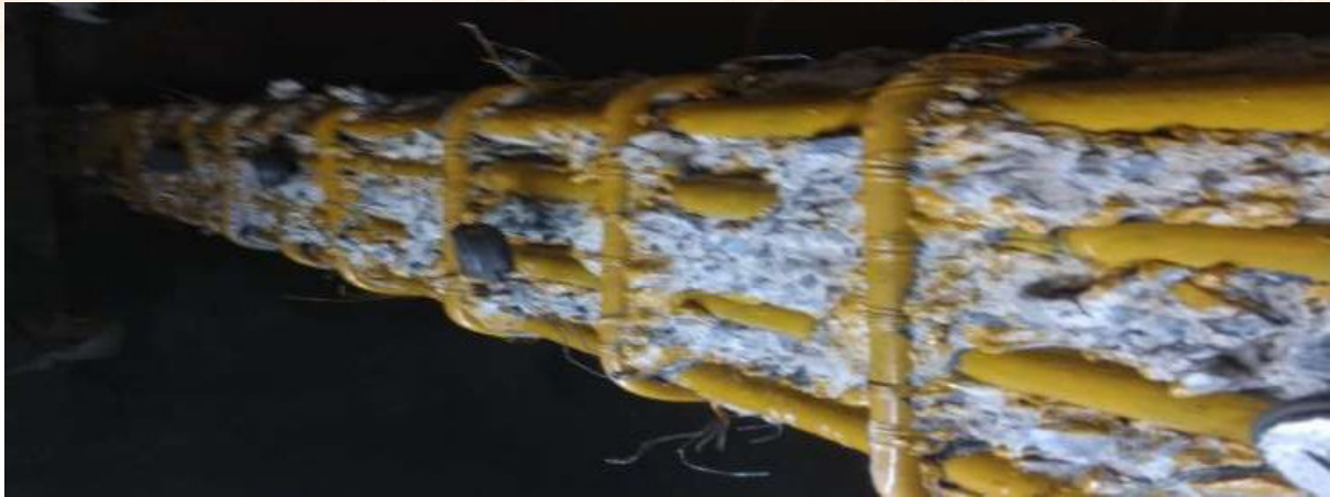
Step-4:- Application of Corrosion Inhibitor on RCC Beam at Nehru Nagar Flyover (RoB)
