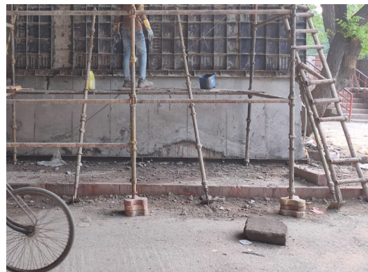
Step-5:- Shuttering work on Pier at Nehru Nagar Flyover (RoB)
