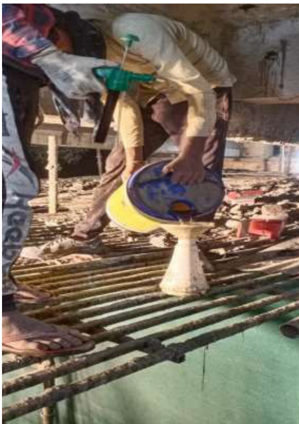
Step-4:- Application of Corrosion Inhibitor on RCC Beam at Nehru Nagar Flyover (RoB)
