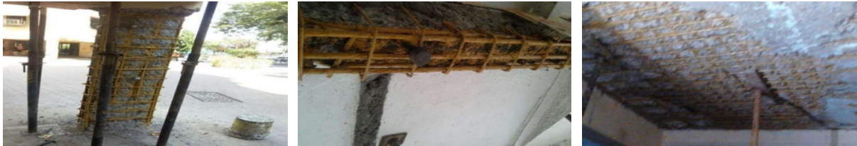
Fig: - Corrosion treatment of Column, Beam and Slab
