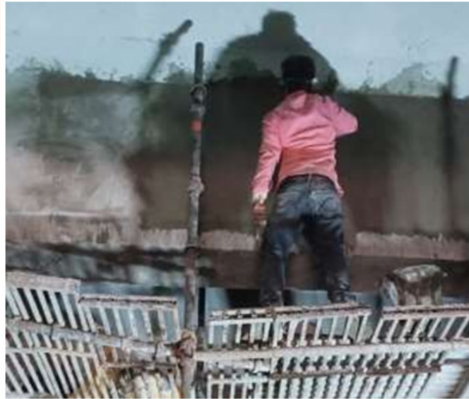
Step-4:- Plastering with PMM on RCC Girder at Nehru Nagar Flyover (RoB)
