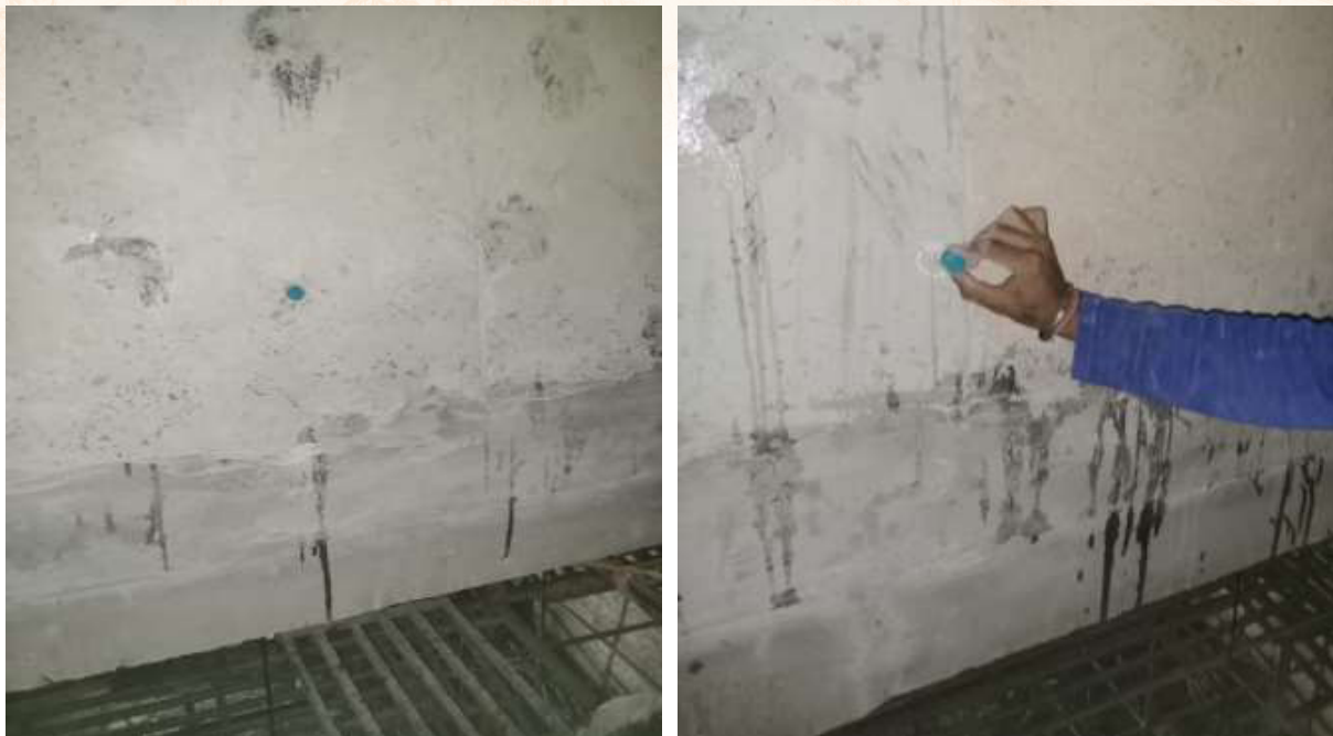
Step-6:- Fixing Corrosion Inhibiting Caplet on RCC Girder at Nehru Nagar Flyover (RoB)
