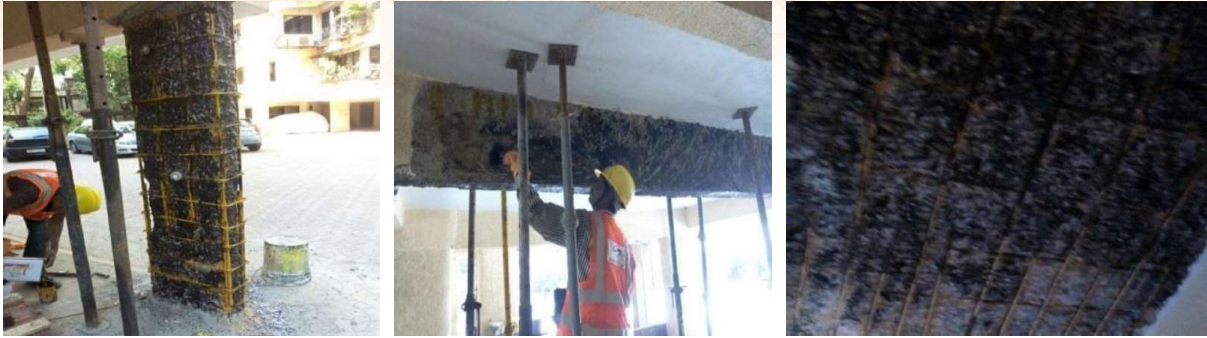
Fig: - Bonding coat on Column, Beam and Slab
