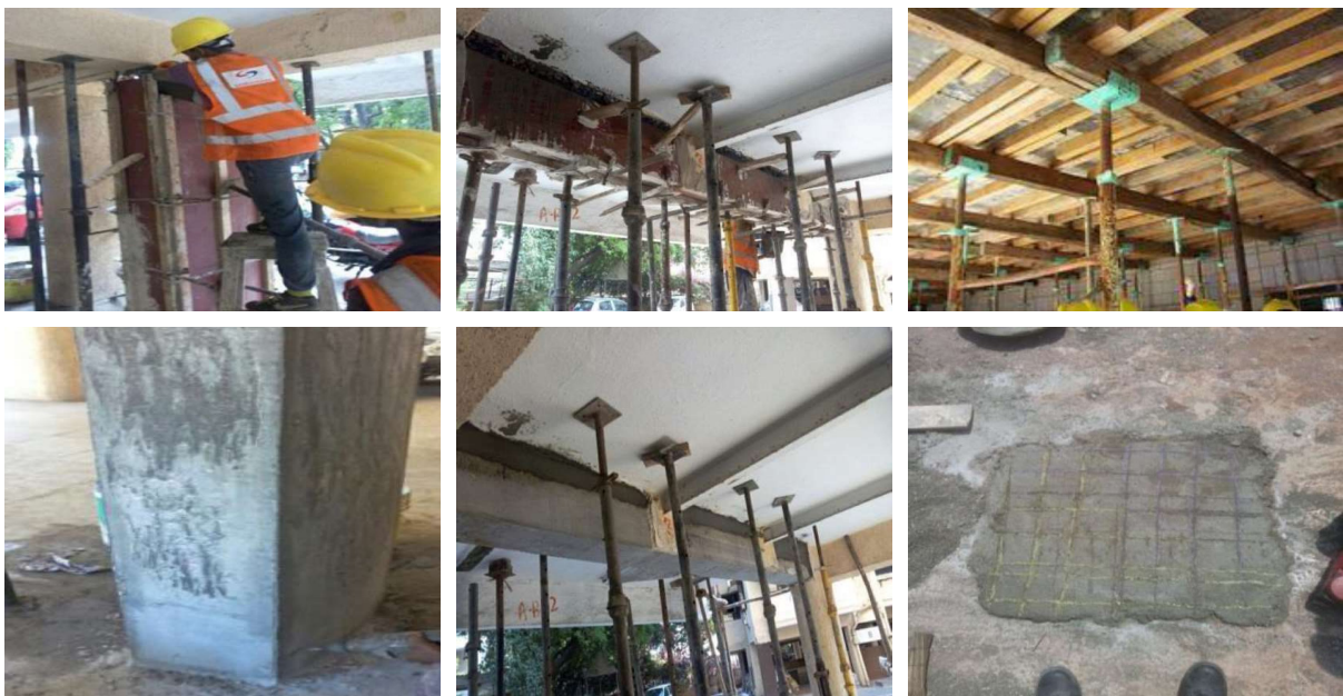
Fig: - Micro Concrete work on Column, Beam and Slab
