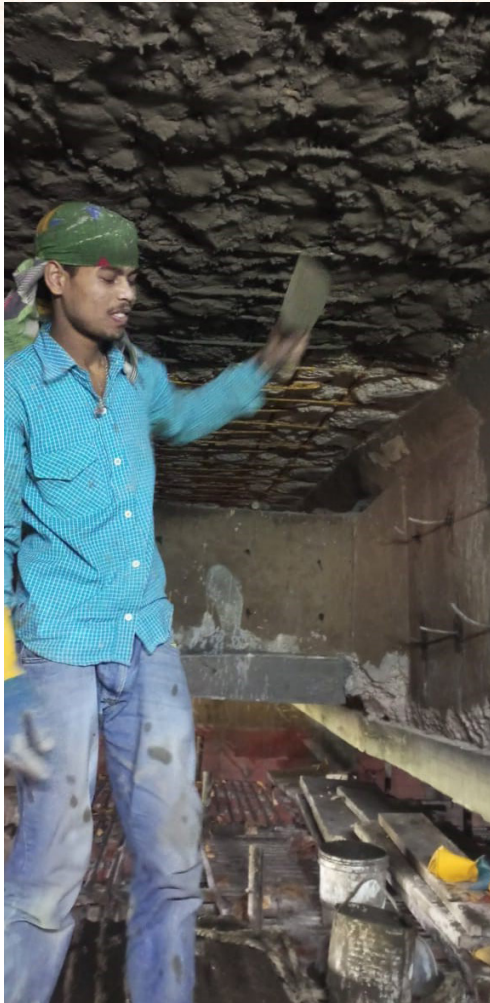
Step-3:- Application of Bonding Coat on RCC Girder at Nehru Nagar Flyover (RoB)
