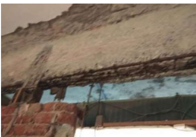
Fig: - Corrosion treatment of Column, Beam and Slab
