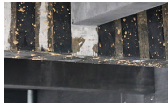
Fig: - Sand pasting on Carbon Fiber
