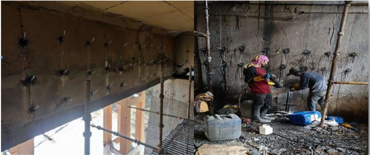
Step-7:- P/F Carbon Laminate on RCC Girder at Nehru Nagar Flyover (RoB)
