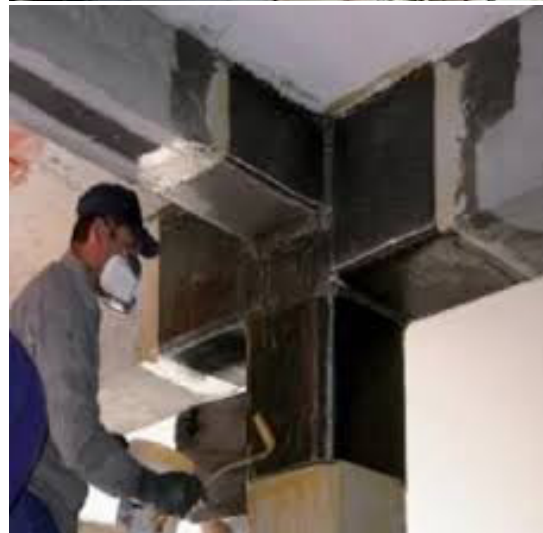
Fig: - Cutting & Fixing of Carbon Fiber on Column & Beam
