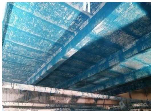
Fig: - Application of Carbon Fiber on RCC structure
