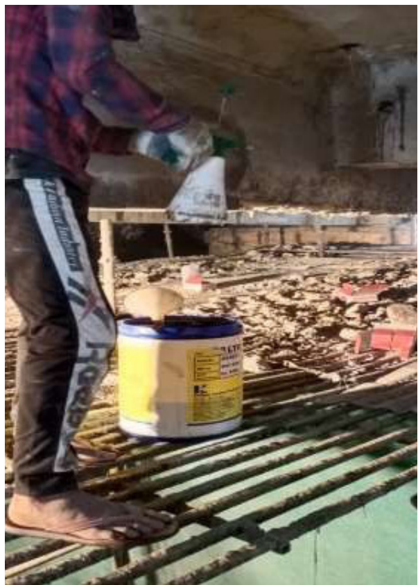
Step-4:- Application of Corrosion Inhibitor on RCC Beam at Nehru Nagar Flyover (RoB)
