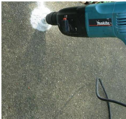
Fig: - Drilling Holes
