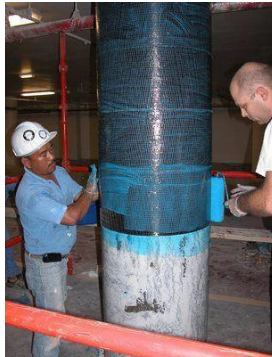
Fig: - Application of second coat of Saturant on Carbon Fiber
