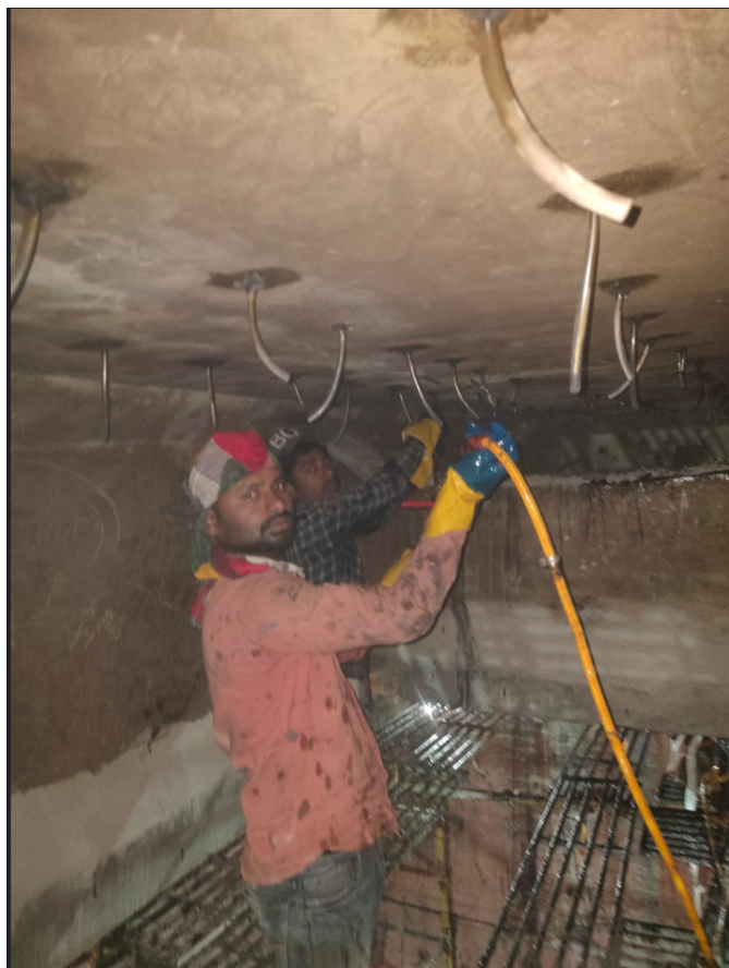
Step-5:- Fixing of Nipples on Deck slab at Nehru Nagar Flyover (RoB)
